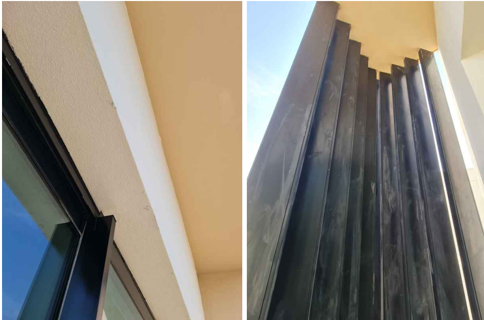
Paint poor finish
