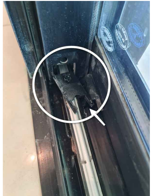
Channel track damage
